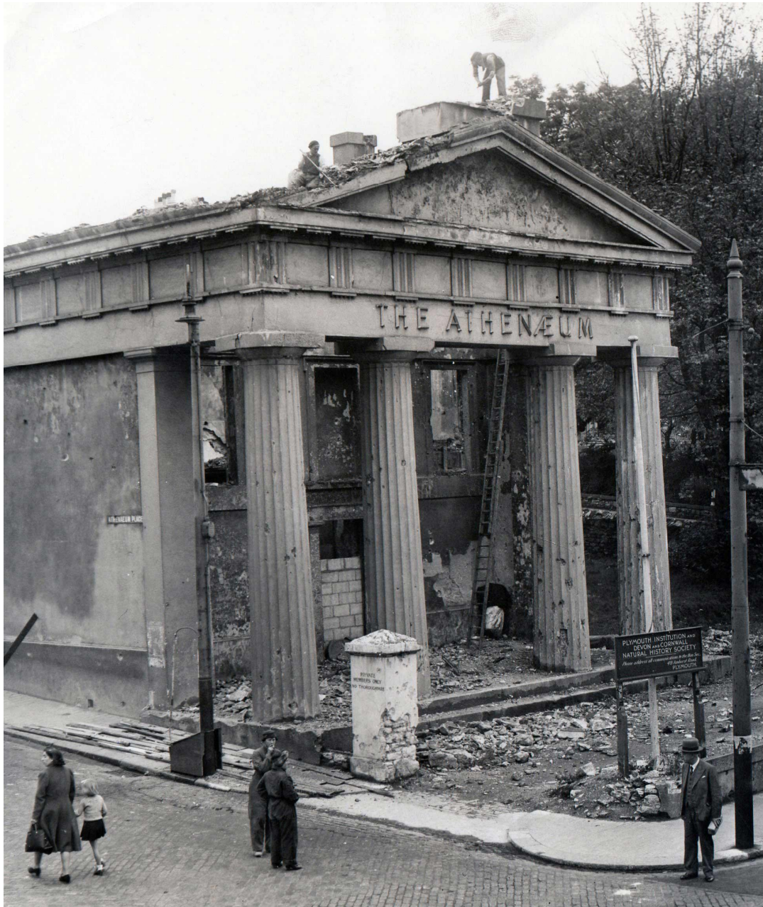
This photograph shows workmen making the Blitz-damaged Athenaeum safe
