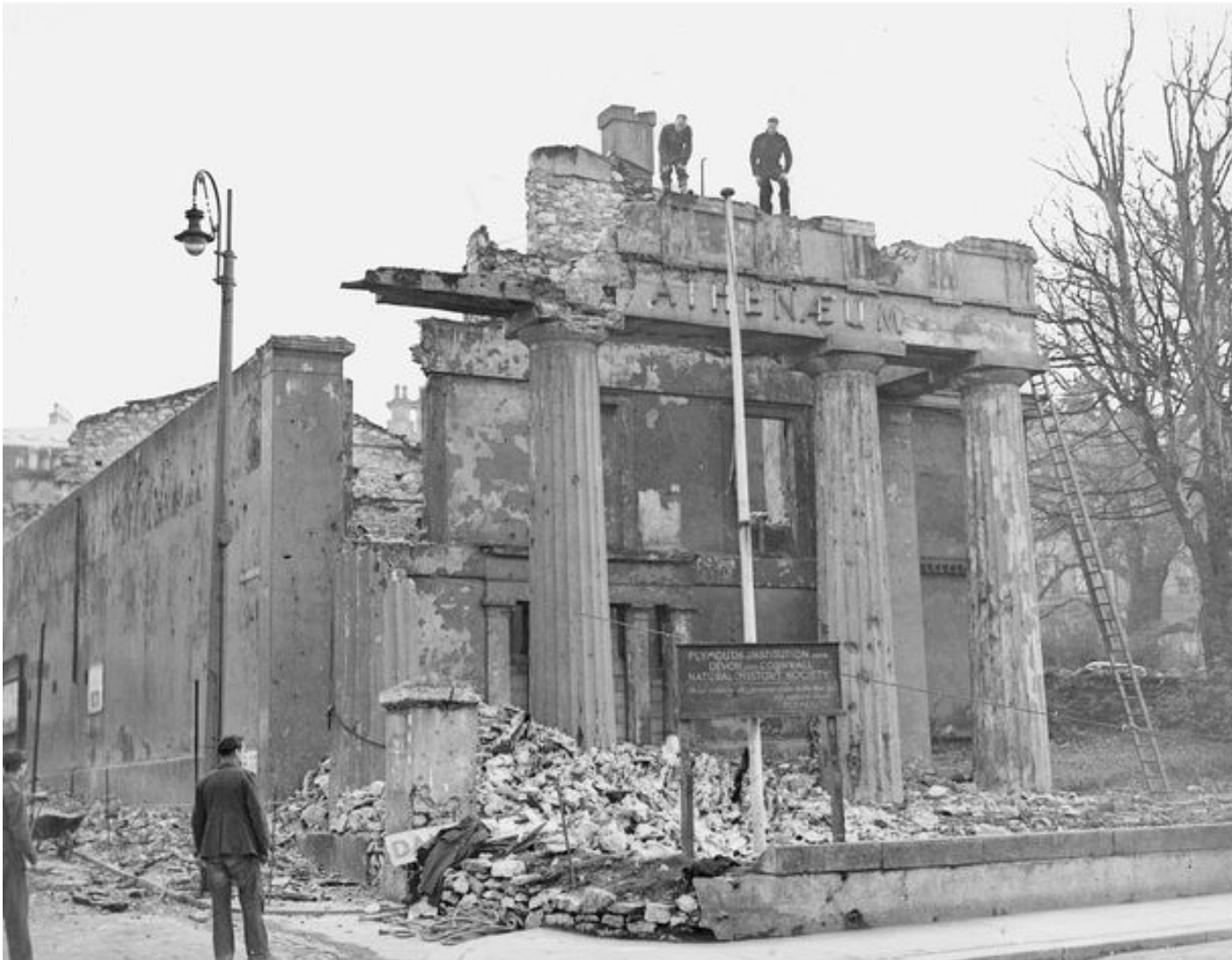
This photograph showing workmen on site at the Blitz-damaged Athenaeum. The upper half of the easternmost of Foulston's Doric columns has been taken down.
