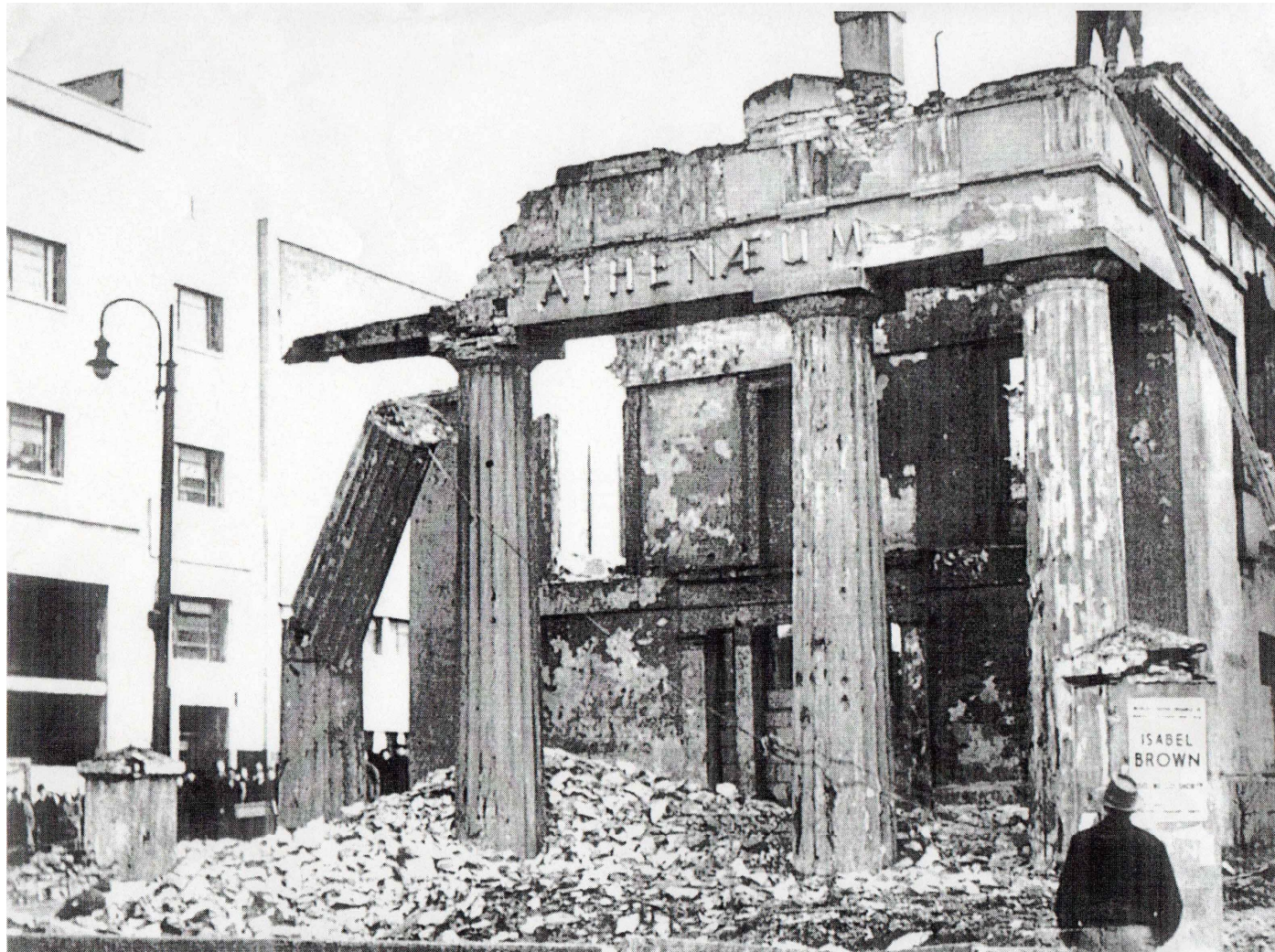
This photograph shows crowds watching the removal of the portico at the Blitz-damaged Athenaeum
