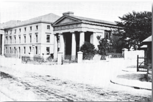
Extentions were added to the building in the 19th and early 20th Centuries
